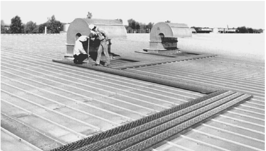
FIGURE 14-16 Roof accessories/walkways.
