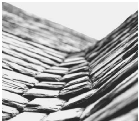
FIGURE 9-3 Textured slate roof.
