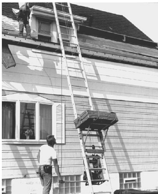
FIGURE 4-15 Typical platform hoist.
