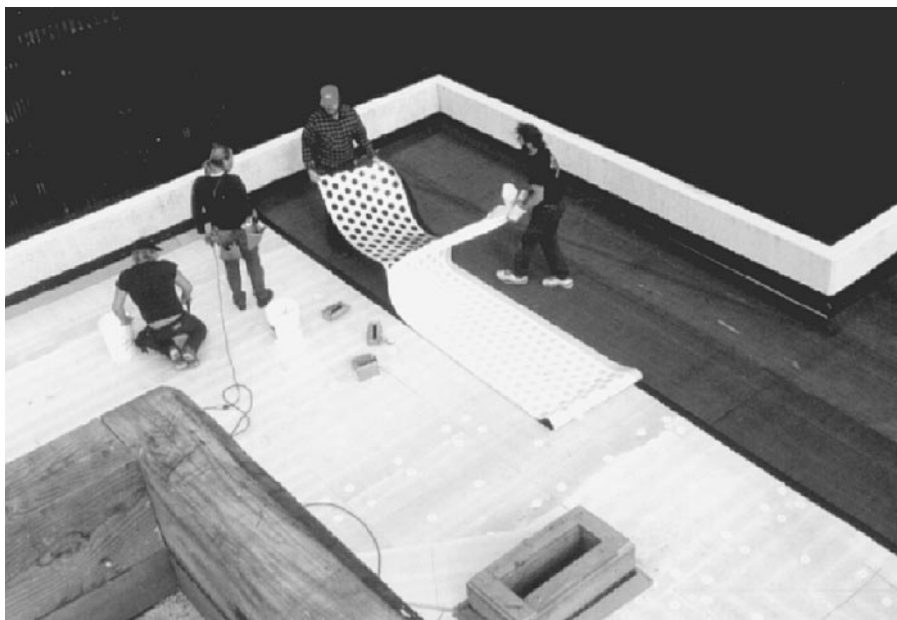
FIGURE 6-1 A single-ply installation.
