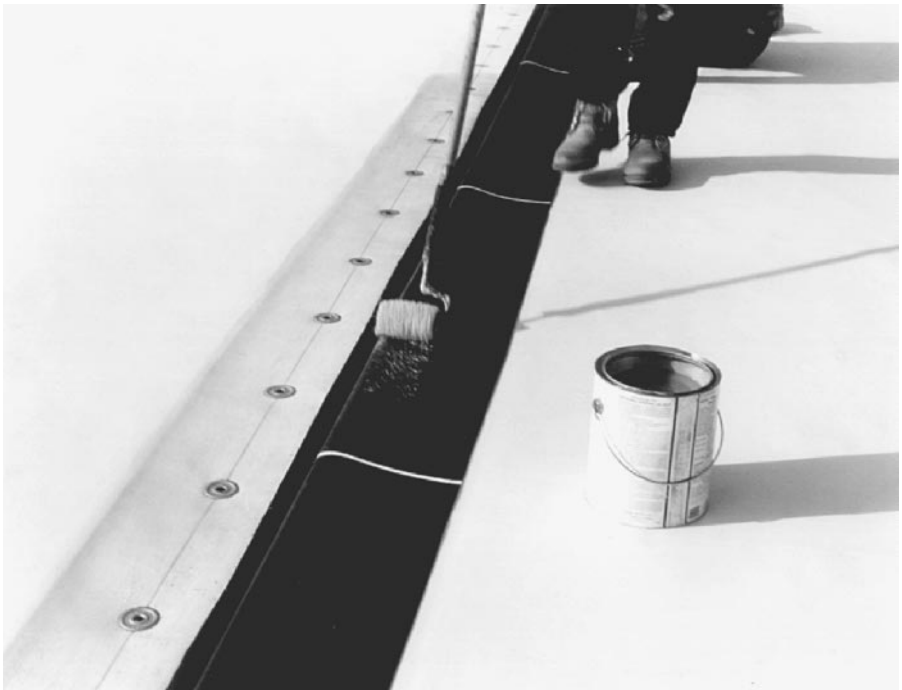
FIGURE 6-2 Apply adhesive on a fully adhered EPDM roof.
