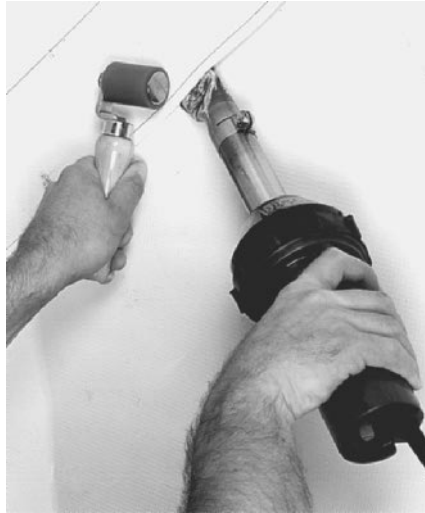
FIGURE 6-13 A hand welder in use.
