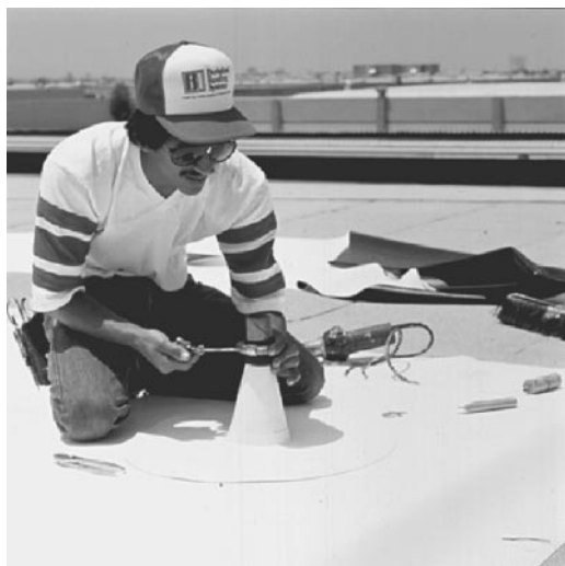
FIGURE 6-14 Making an adjustment on a hand welder.
