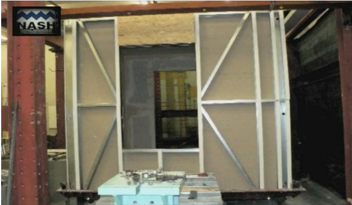
Figure 1: A New Zealand Light Steel Frame (V.P. Paton-Cole 2010)
